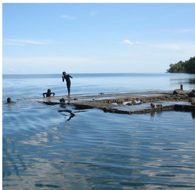
A submerged wharf on Simbo. The island sank nearly one meter during the 2007 earthquake. Photo credit: Matthew Lauer
